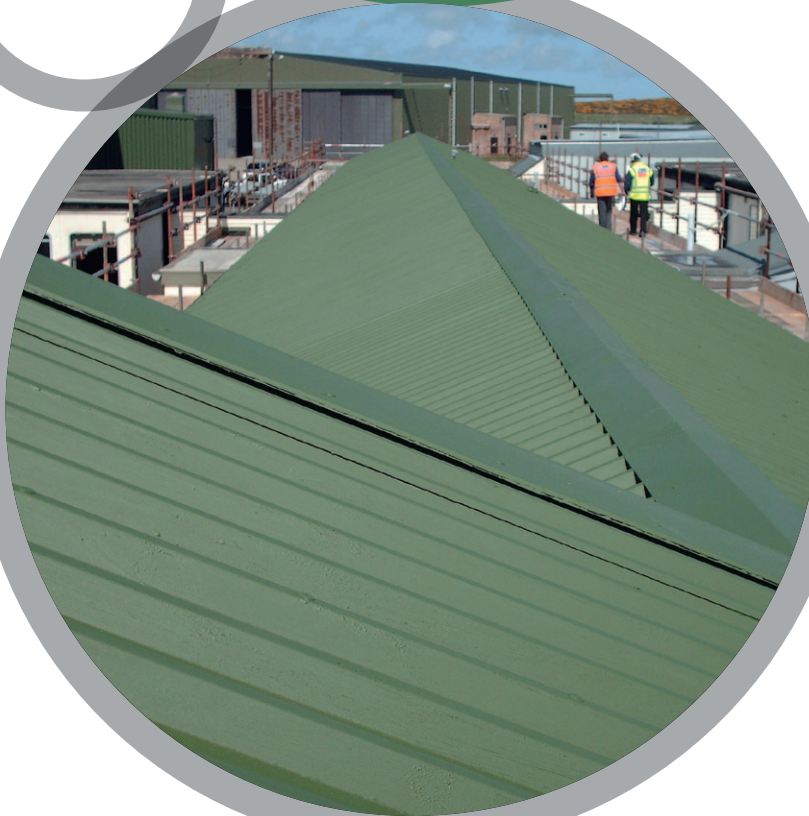
Fully Encapsulated Roof Repair & Protection System
